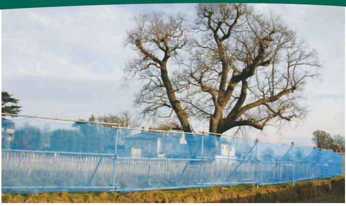
Substantial fencing has been used according to BS 5837 Trees in relation to construction, to protect the roots of this old pollard estimated to be 500 years old.
