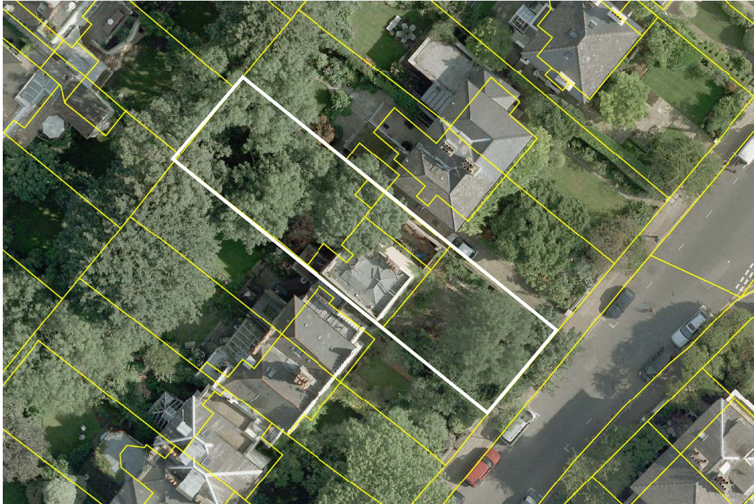
2007 Prior to construction of basement
